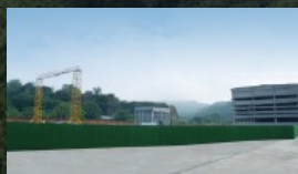
Ground Integrated Test Center
