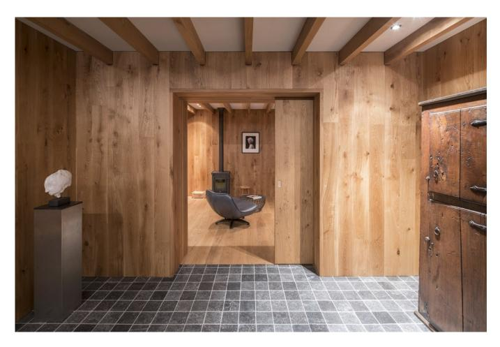
Boom explains: "We designed every space with 1.80 meters – plank size – as our base unit, looking to create a perfect rhythm and interplay of lines. That's easy enough on the drawing board, but very difficult to get right in practice. The dimensional stability of the **Hakwood** planks played a vital part in getting it just right."
